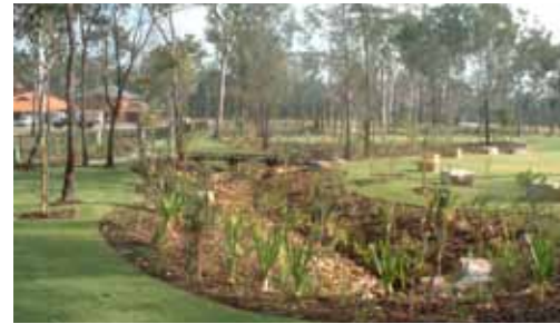
Water management swale
